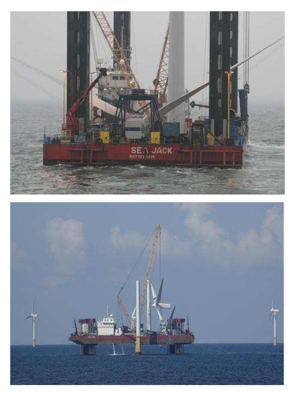
**Figure 6**. Construction activities in PAWP: preparations for hoisting a turbine. Building PAWP took place while OWEZ was already fully operational and while T-1 seabirds surveys (see main text) for OWEZ were conducted. Photos: Hans Verdaat, IMARES (top) Kees Camphuysen, NIOZ (bottom).
