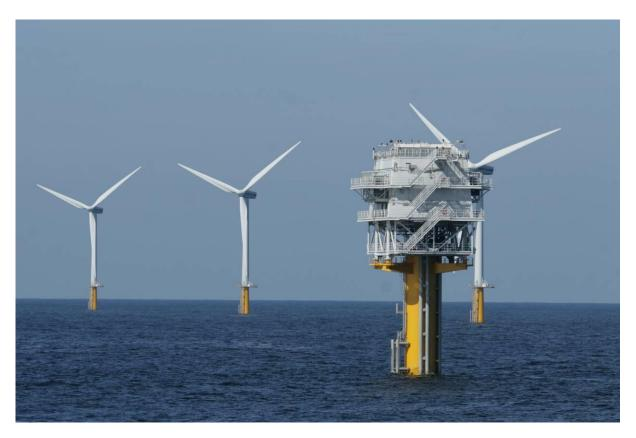
**Figure 3**. Transformer platform and three of the 60 turbines of PAWP. The PAWP turbines are smaller, but placed closer together than the OWEZ turbines. Note that both the PAWP transformer platform and the OWEZ metmast offer a platform for roosting seabirds, such as cormorants and gulls. Photo: Hans Verdaat, IMARES.
